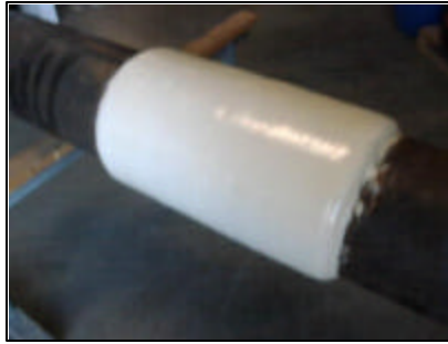
Fig. 8 – Finished repair with 34 layers of Aquawrap® G-05.
